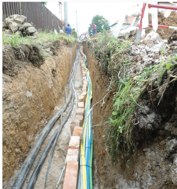
Laying down cables in a trench
