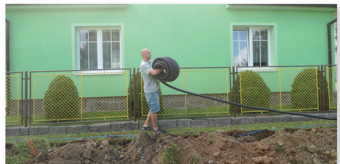
Laying down protective hosing
